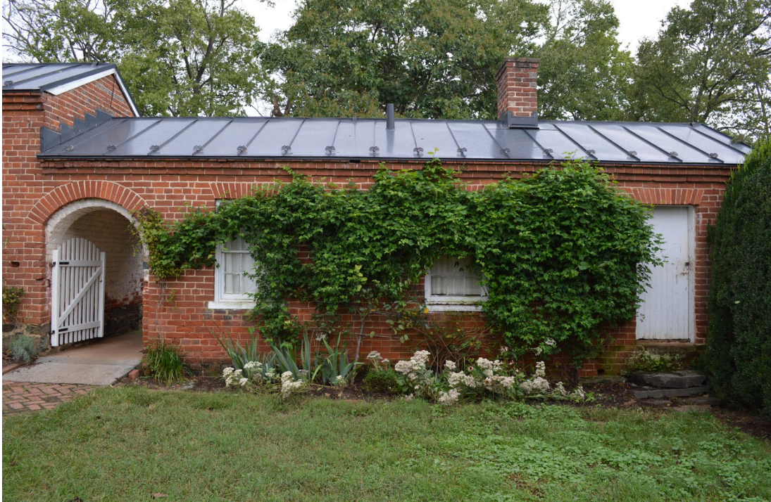
Figure 12. Addition 2, south elevation; east doorway converted from a window; two left bays fronted the heated space, likely to accommodate slaves.
