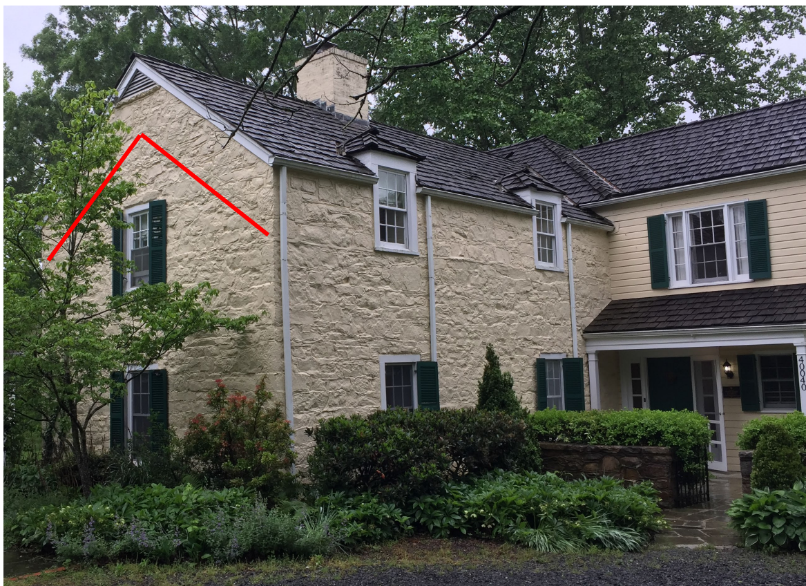
Figure 6. Hamlet Duplex, north and east elevations (on the left); incorporated as a wing to the former Emmet House, now the Inn at Oatlands Hamlet (2018). Raised from 1.5 to 2-stories, dormers added (former gable roofline in red).
