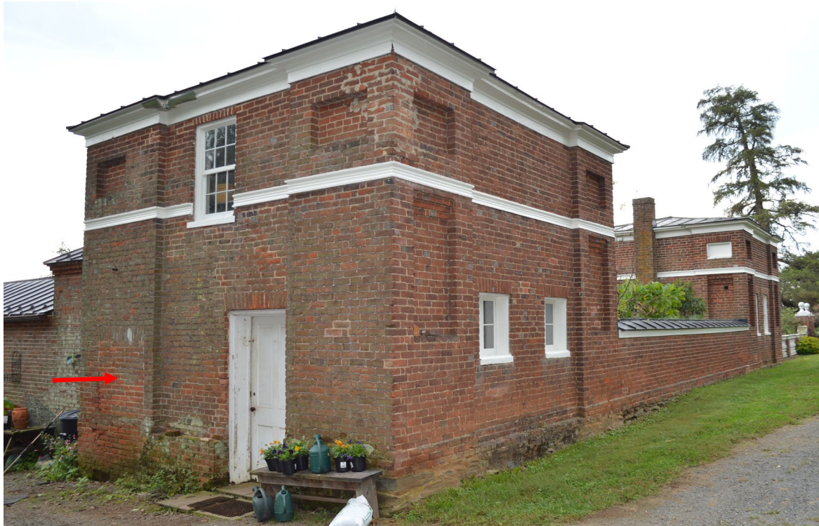
Figure 10. Pavilion north and west elevations (2018); two doorways in the north façade are original but have been altered (location of infilled doorway indicated by red arrow).
