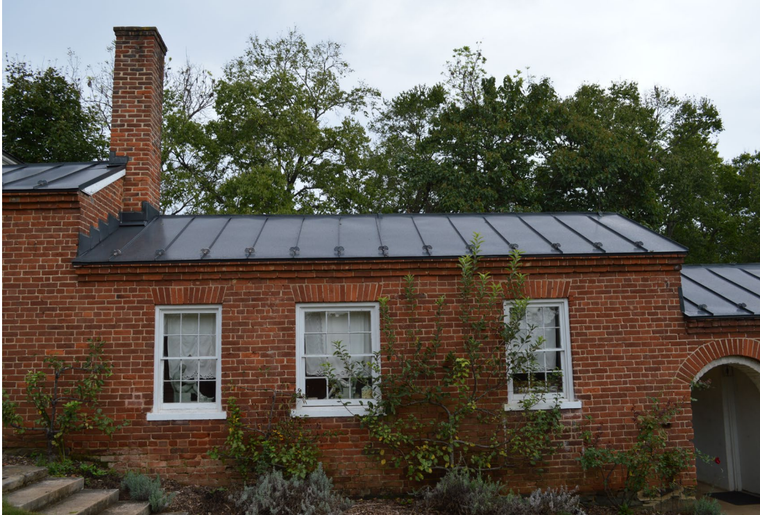
Figure 11. Addition 1, south elevation; center window originally was a doorway; two left bays front the heated space, which likely accommodated slaves.
