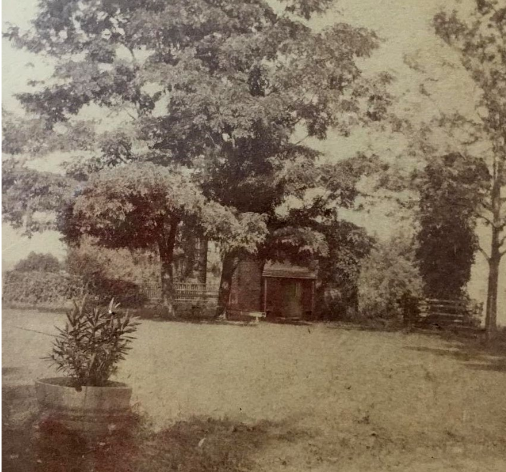
Figure 8. Undated photo of the structure (non-extant) identified as the Garden House on the 1923 plan, viewed from the west.
