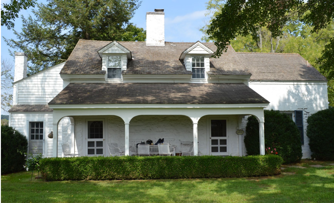
Figure 5. Little Oatlands Duplex 2, south façade (2018); dormers, porch, and wings added.
