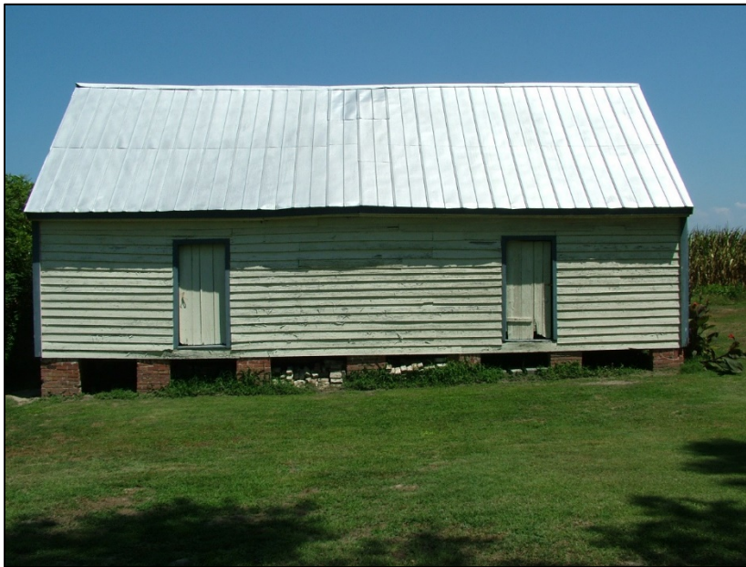
Figure 3. The frame quarter at Four Square plantation, in Isle of Wight County, was erected in two phases, dendro-dated to 1789 (right) and 1830 (left).
