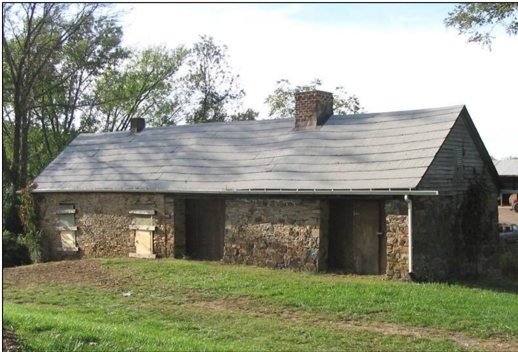
Figure 1. The stone Arcola slave quarter, Loudoun County; the two phases of the building's construction were dendro-dated to 1813 (left) and 1845 (right).
