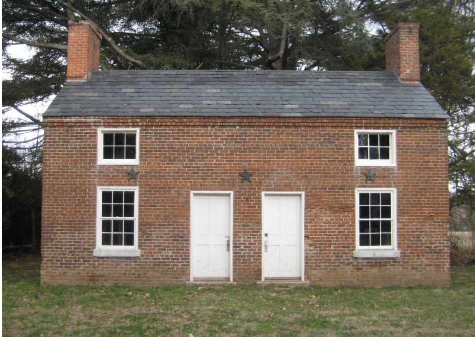
Figure 1. Sherwood Forest kitchen-laundry-quarter, south elevation (2015).
