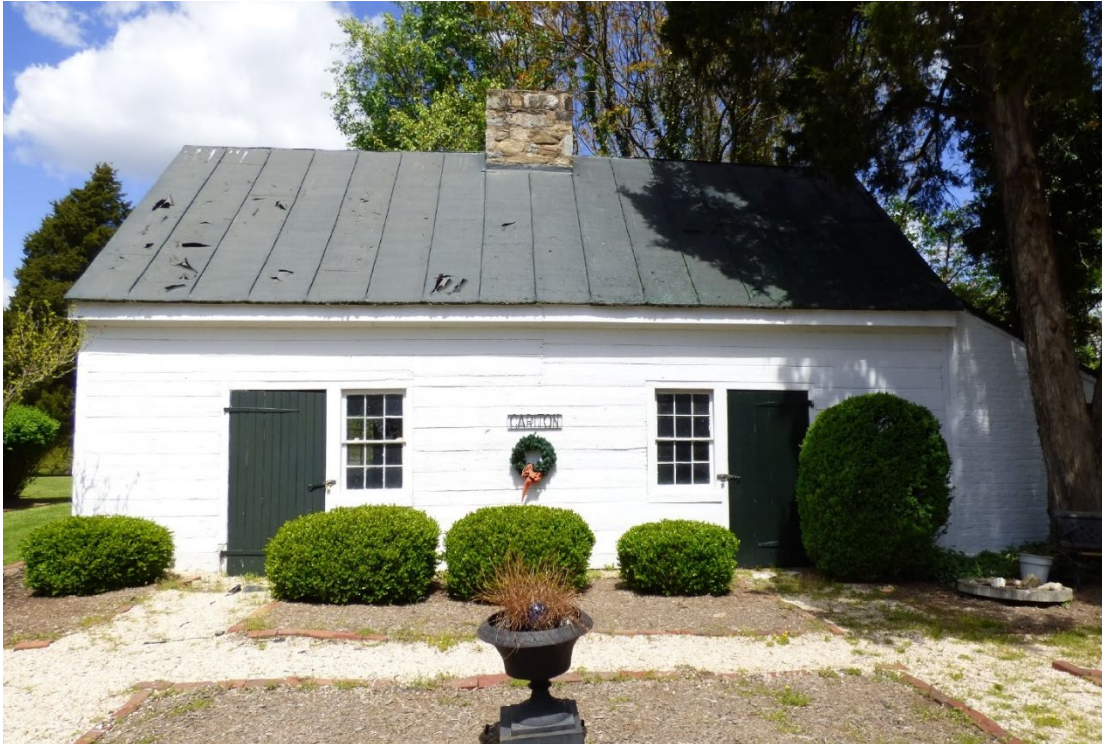
Figure 6. Carlton duplex, south elevation (2015).
