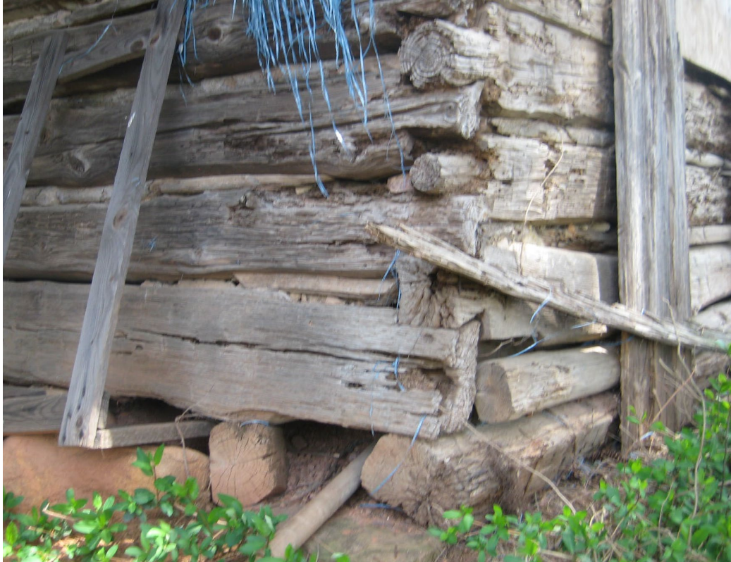
Figure 15. Sanford-Burgess cabin, detail of log corner notches (2015).
