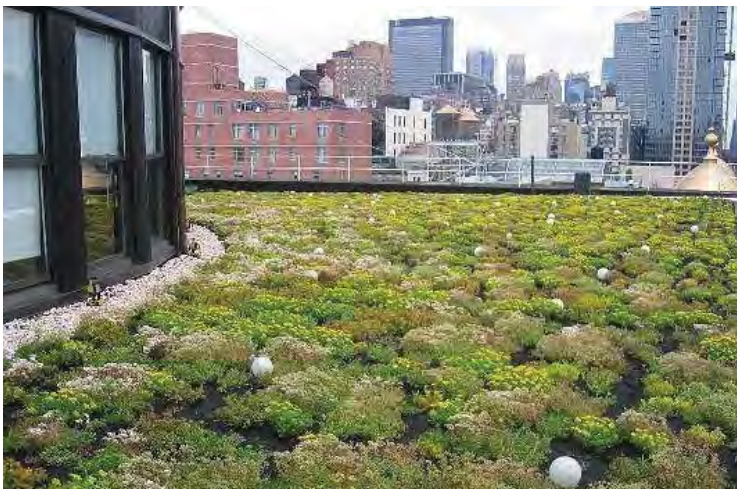
View of an extensive green roof made of low growing vegetation.
