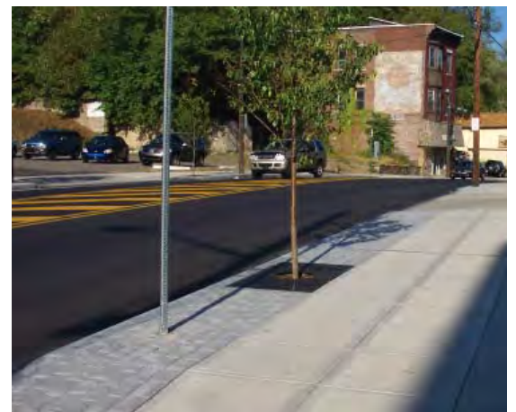
Existing conditions of a sidewalk in Providence Square. This technique can be utilized throughout the neighborhood to tie it together but utilize infiltration bed and permeable pavers.
