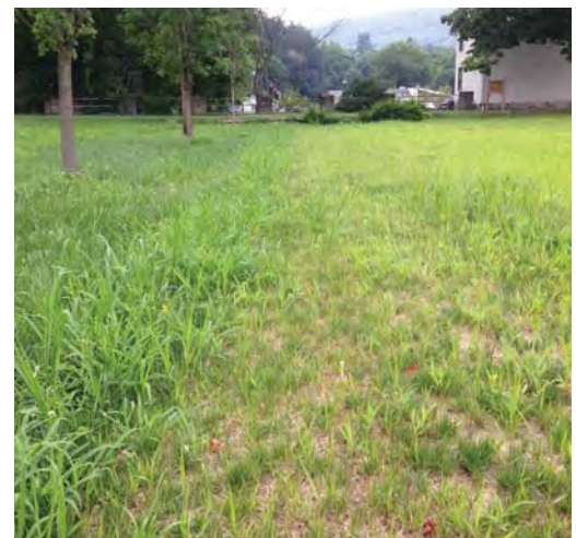
Hillside Farms in Shavertown, PA used a grid system filled with grass for an overflow parking area instead of traditional asphalt. The grass fits in with the farm atmosphere. (Picture above is 1st year of growth.)
