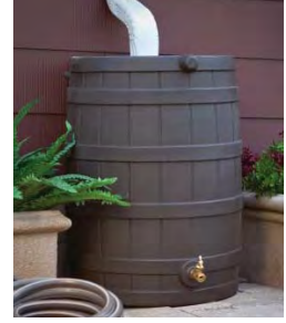
A rain barrel attached to downspout.
