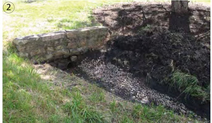
Water from the drive is piped to the open space, runs into Meadow Brook and eventually to Lackawanna River.
