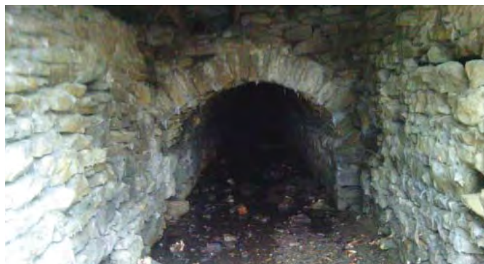
Meadow Brook: example of historic construction.
