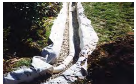
A french drain before it is covered with dirt.
