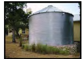
Above ground cistern.
