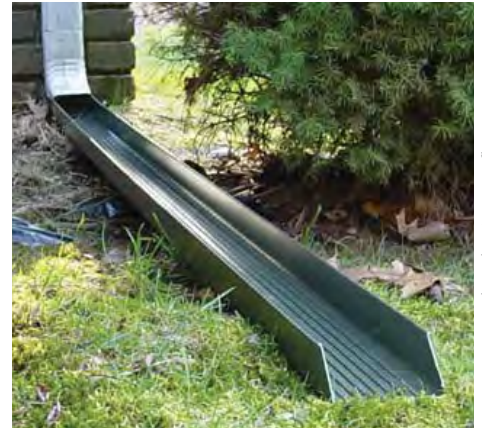
Example of a downspout that is disconnected and directing water away from the building into a lawn area.
