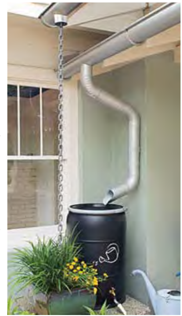
A downspout being directed into a rainbarrel.
