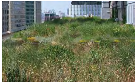
Data collected from Chicago's City Hall's green roof indicate that the roof not only reduces stormwater runoff by 50 percent, but significantly reduces energy use and saves the City approximately $5,500 annually on heating and cooling expenses 22
