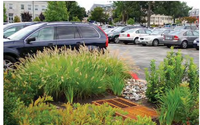
Raingarden located next to a parking lot. The overflow is sent into the catchbasin.
