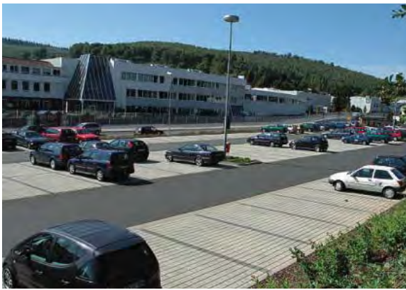
Pervious pavers replace the parking spaces.
