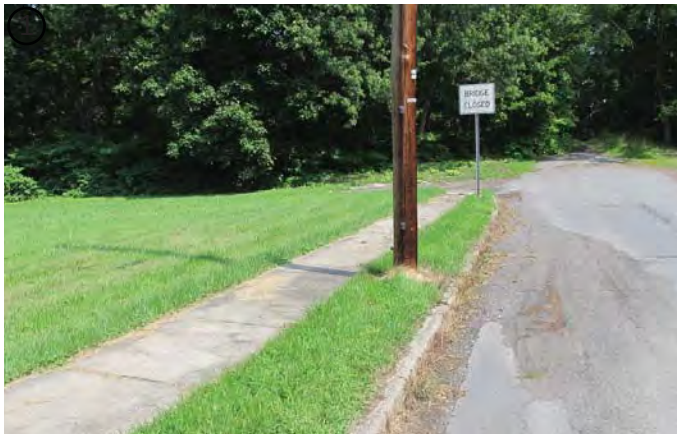
Water currently runs along the existing curb and into Leggett’s Creek at the end of the road. In this picture, the transported and deposited sediment is visible.
