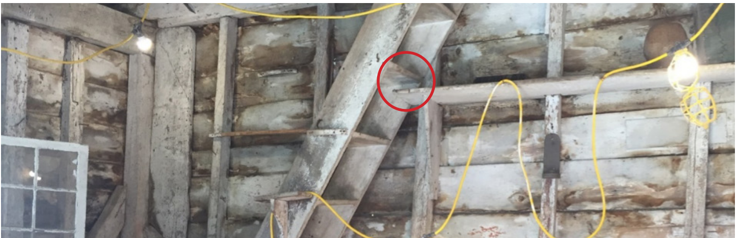
Figure 10. Detail of the northwest section of the north wall, showing the relationship of the stairway and the shelf; the west end of the shelf has an uneven vertical cut, indicating that it was trimmed to allow sufficient space to install the ladder stair (2018).
