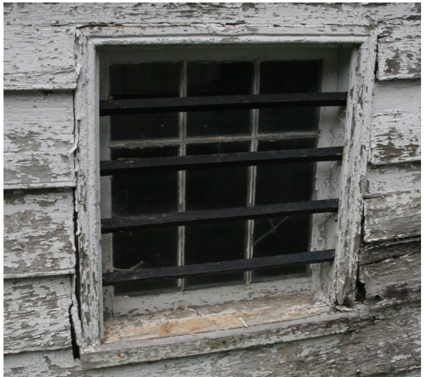
Figure 13. Window with hinged sash and iron bars, east elevation (2018).
