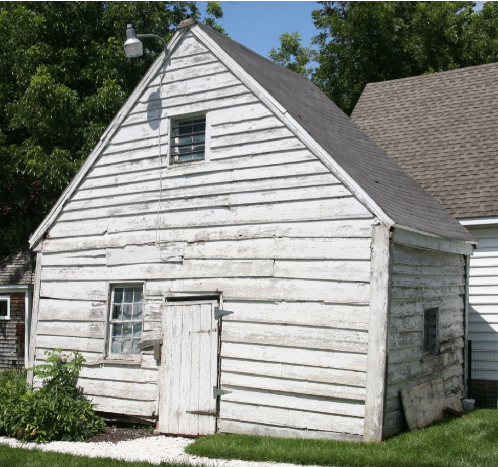
Figure 2. South-facing façade of the Bayly outbuilding (2018); doorway and windows are later insertions.
