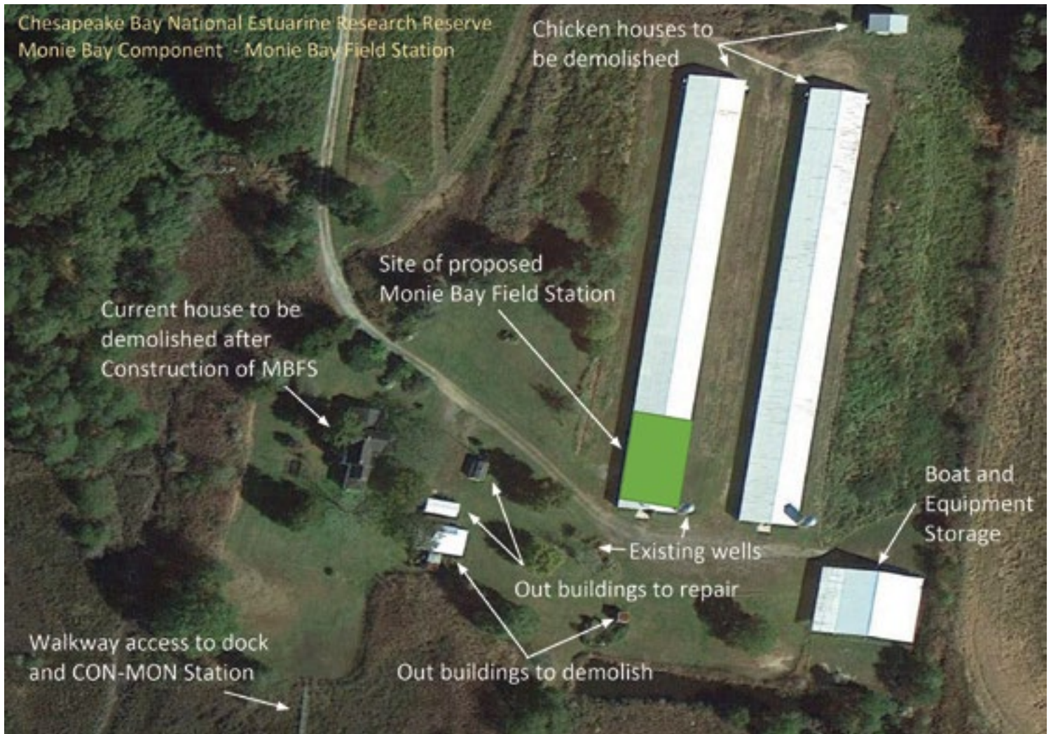
Overview of existing site conditions at Monie Bay Field Station (DNR)
