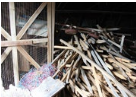
Salvaged lumber from deconstruction may be reconfigured for use in finish trim
