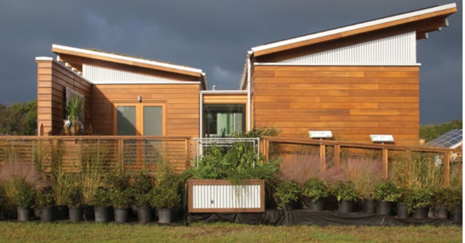
University of Maryland's WaterShed, 2011 Solar Decathlon Entry
