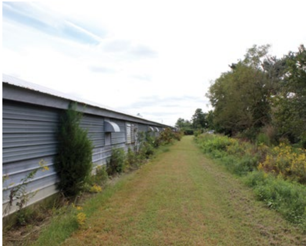
CLOCKWISE FROM TOP: 52,740 sf of corrugated galvanized steel is available from existing chicken sheds on site; Additional view of chicken shed on site; Existing grain silos on site may be re-purposed
