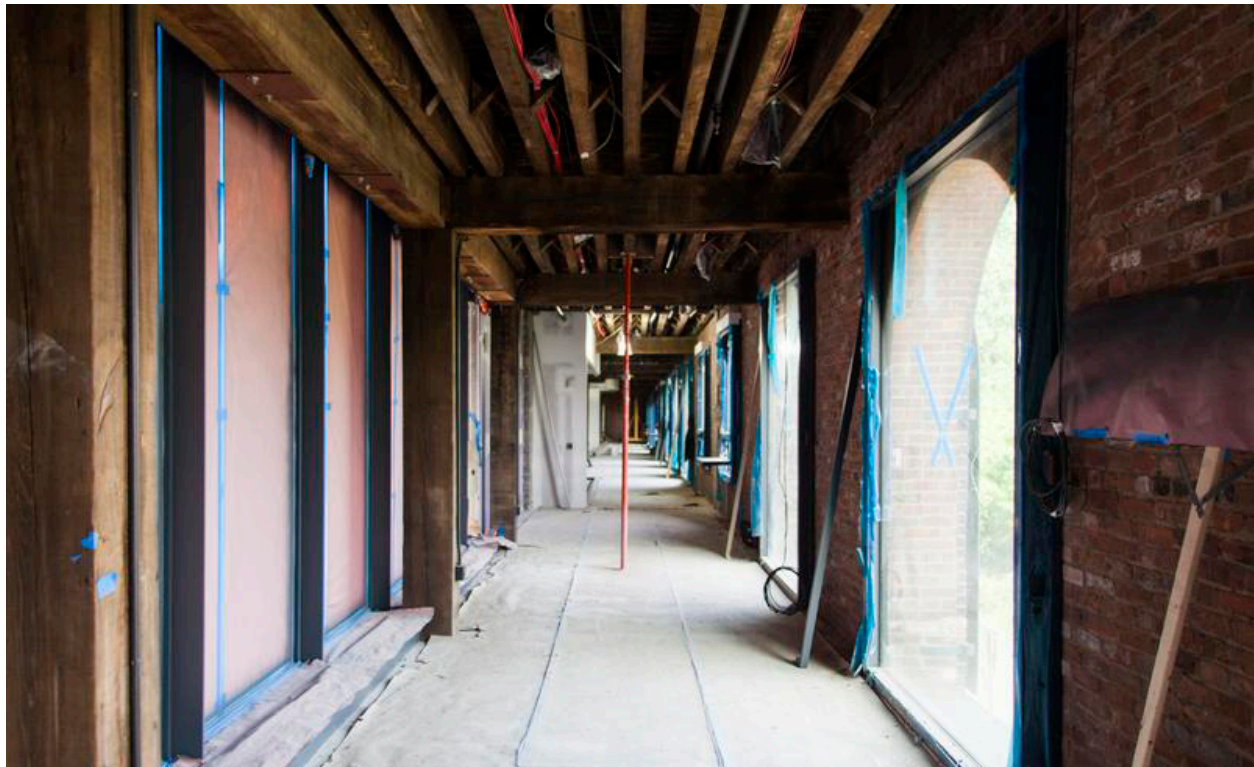
Image Above: New Helical Mini Piles (Silman) Image Below : New rectangular glass windows over existing arched openings
