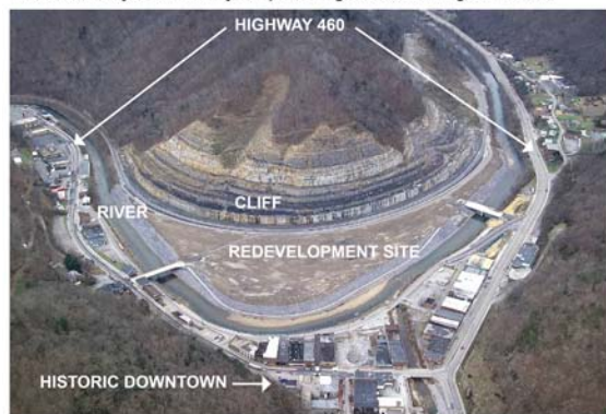
AERIAL PHOTOGRAPH SHOWING THE RELATIONSHIP BETWEEN THE HISTORIC DOWNTOWN AND THE REDEVELOPMENT AREA WITH CLIFF
