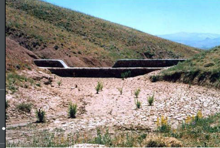
Check Dams - Gabion
