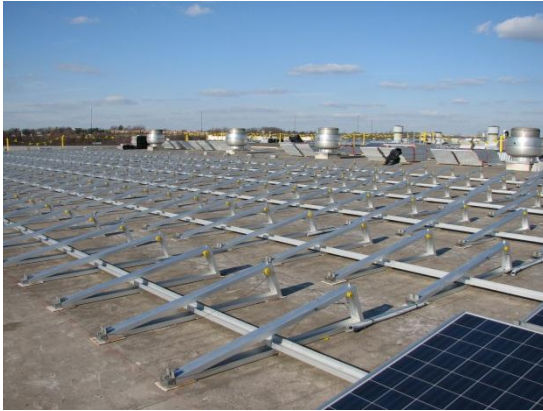
NMWDA – Installation of Racks for Ballasted Rooftop Mounts
