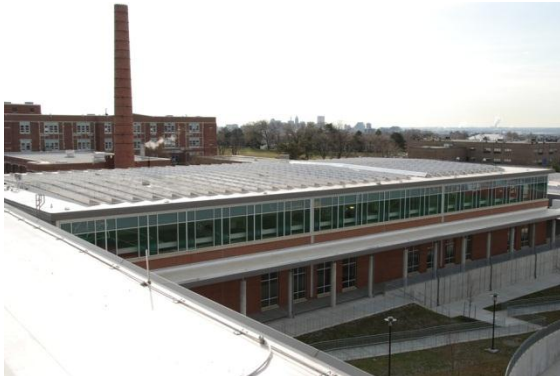
Coppin State University – Ballasted Rooftop Mount
