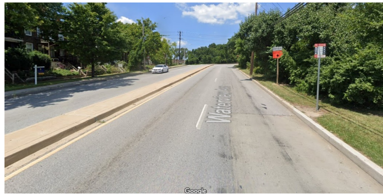
Figure 5-3. Street view of the Waterview Avenue northbound bus stop. Inclement weather and nighttime conditions create further challenges for riders using this bus stop. Lack of adequate lighting reduces the visibility of riders who cross the street to access this bus stop. The curb where the bus stop is located has no curb cuts, which poses challenges to access for riders who rely on mobility aids or those with limited mobility.
