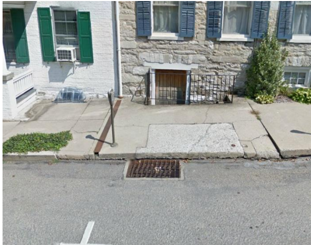
Figure 2 – Example stormwater inlet along Main Street in Mercersburg. Note the downspout drainage connection to the roadway just to the left of the inlet.
