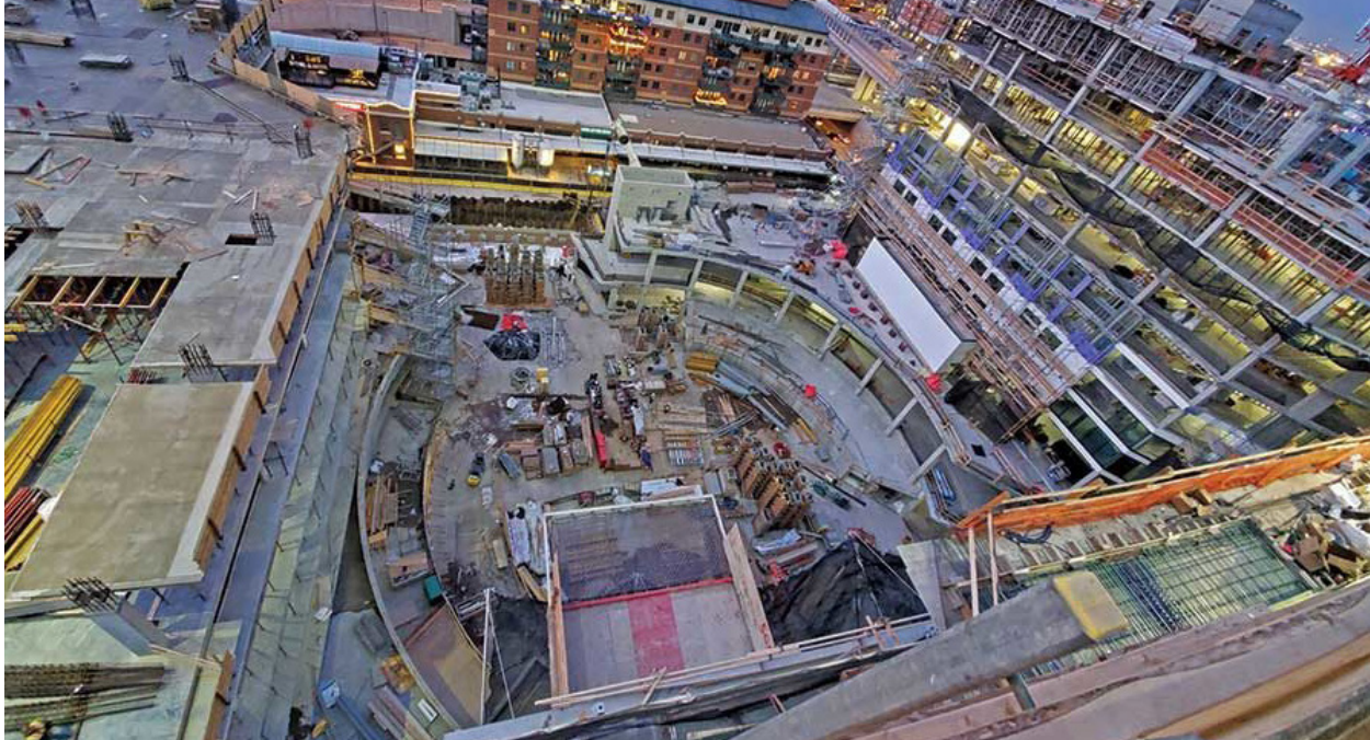
Construction Underway. Courtesy of Engineering News Record.
