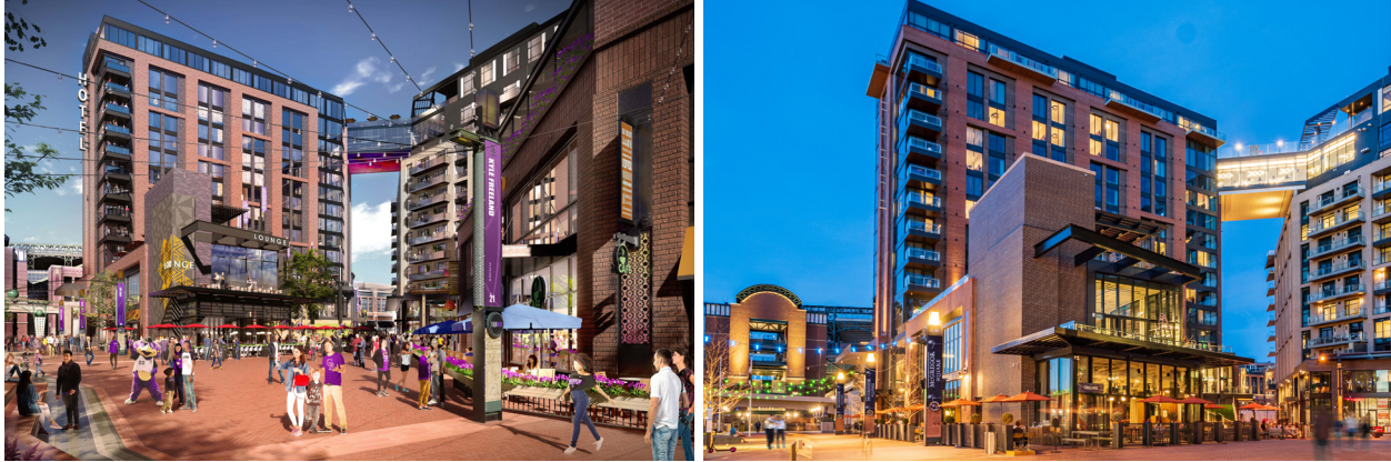
Side-by-side rendering (L) and finished product (R) of the sky-bridge connecting the condo & hotel towers. Courtesy of Stantec.
