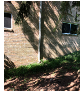
Figure 9 Community garden downspout
