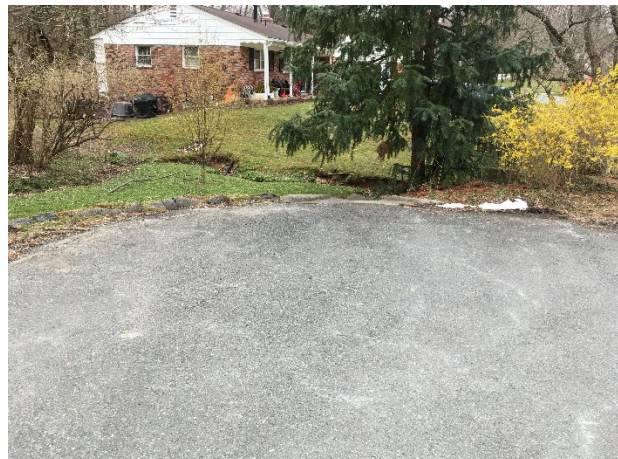
Figure 2: Opportunity to remove impervious area in a cul-de-sac and replace with a bioswale/channel stabilization
