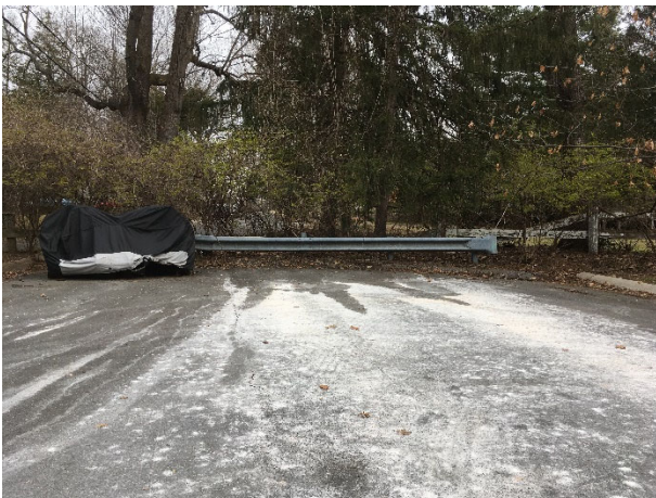
Figure 1: Impervious removal and bioretention installation
