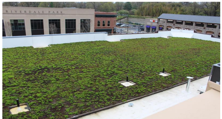
Green Roof, Riverdale Park Station
