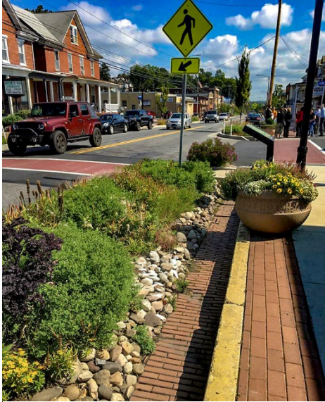
Figure 7: Lemoyne Borough native plant rain gardens. Photo courtesy of Kasha Griva, Lemoyne Borough
