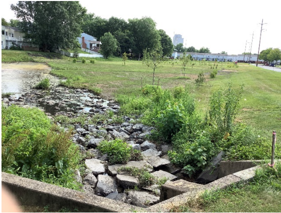
Figure 6: Retro-fitted basin constructed by the Borough to capture drain from downtown and residential sectors. Photo courtesy of Roger Ciecierski, Mechanicsburg Borough
