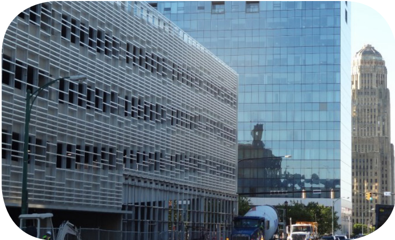
View of Parking Garage from South Elmwood Ave.
