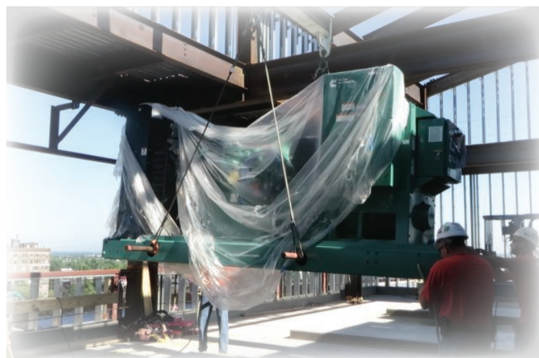
Penthouse generator being installed
