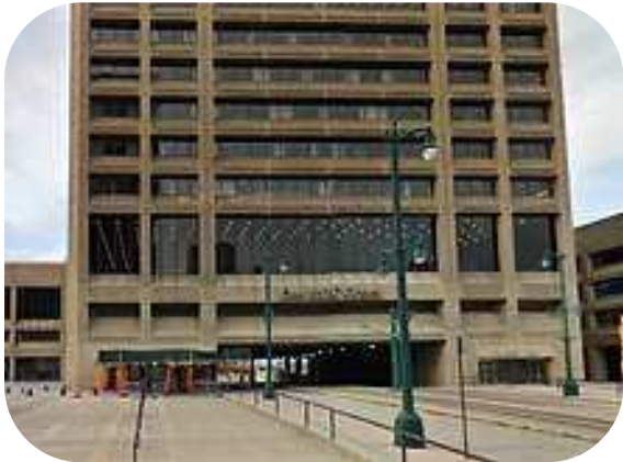
Plaza Before Renovation
