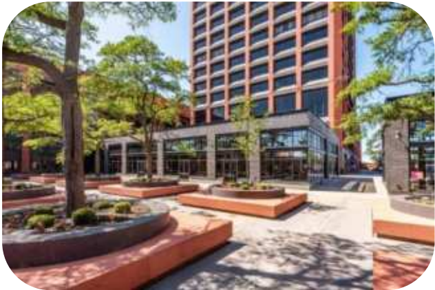
Plaza After Renovation
