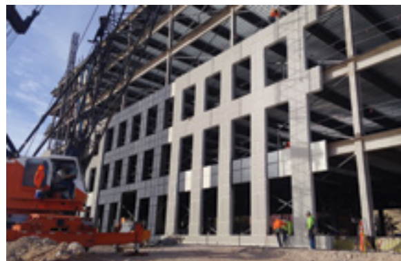
Two Summerlin Precast Panels
