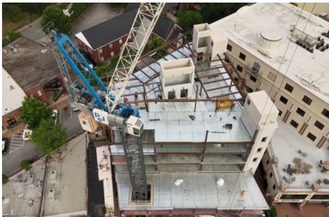
The crane that was used for construction
