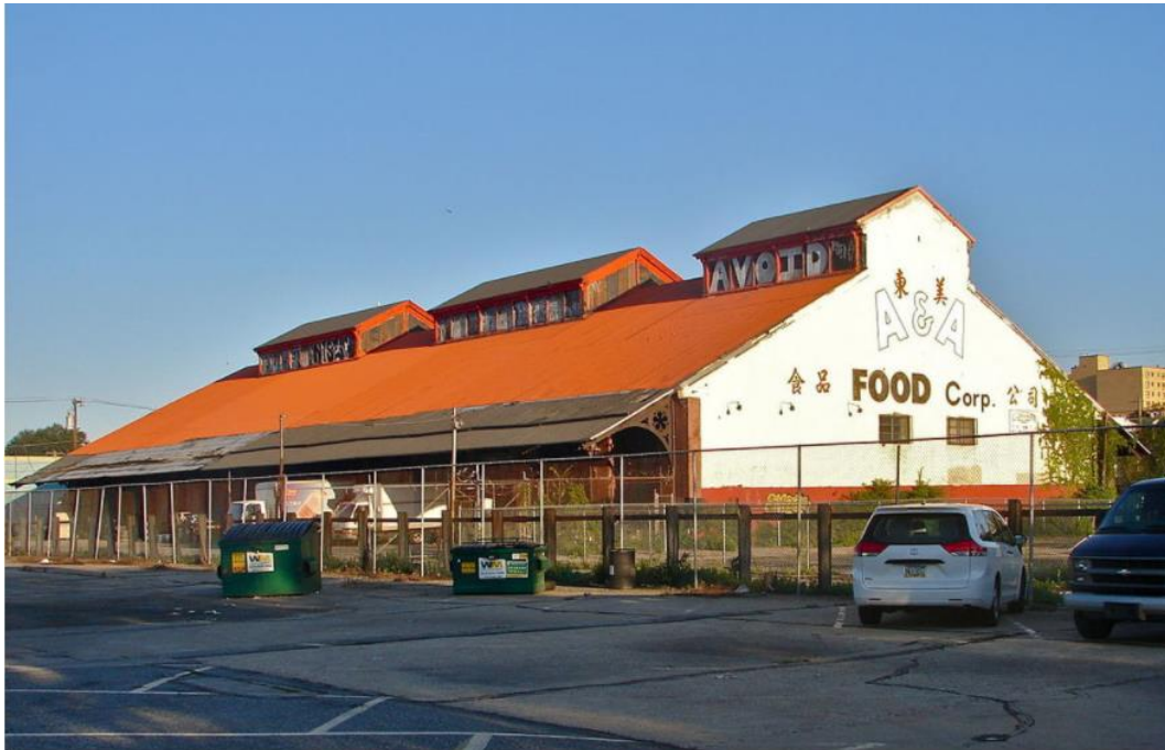
The PW&B trainshed right before construction started on its rehabilitation.
