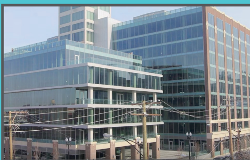
Completion and Turnover
