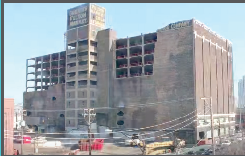
Tearing Down the Façade
