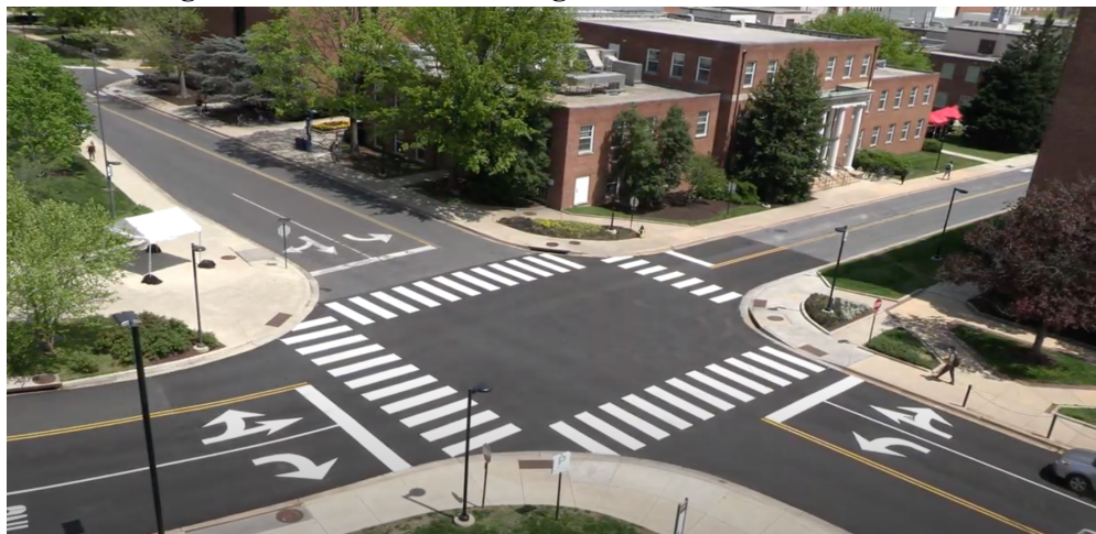
Figure 16: Stadium Drive/Regents Drive Intersection View
