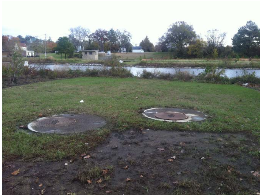
Stormwater baysavers located in the Town of Federalsburg near the Marshyhope
