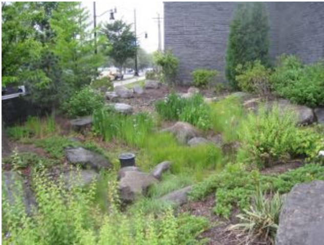
An exemplary display of green infrastructure at The Commonwealth Medical College in the City of Scranton.
