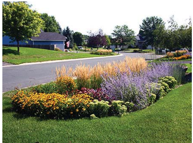
A rain garden implemented in a front yard, next to a roadway can help filter road runoff.
