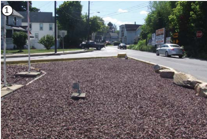
Existing conditions of south side of the memorial consists of gravel and stones.
