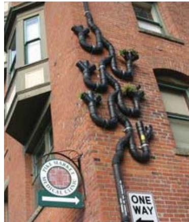
Incorporating the planter into the downspout is another option when room is limited.
