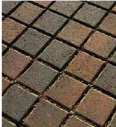
Permeable Pavers: The voids in between the stones allow water to infiltrate through them.
