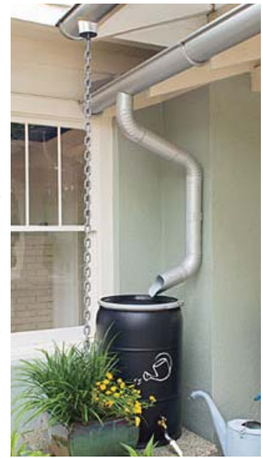
A downspout being directed into a rainbarrel.
