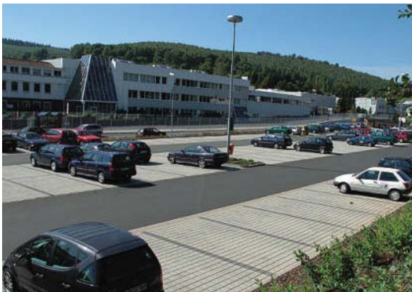
Pervious pavers replace the parking spaces.
