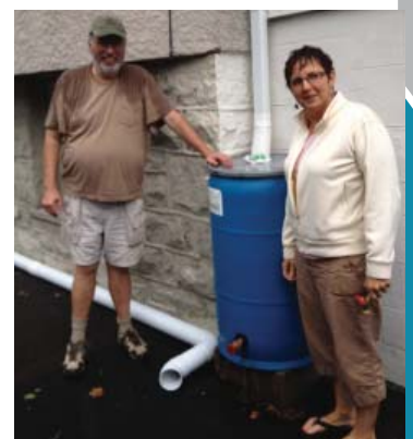
Downspout disconnect with rainbarrel.
