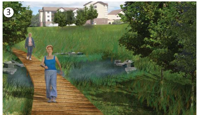
A constructed wetland can be used to handle excess stormwater runoff.
