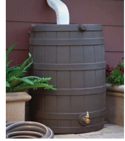
A rain barrel attached to downspout.
