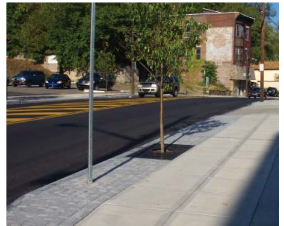
Existing conditions of a sidewalk in Providence Square. This technique can be utilized throughout the neighborhood to tie it together but utilize infiltration bed and permeable pavers.
