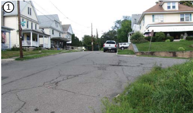
Currently water runs down Belmont street (shown above) passes by the existing site and into a catch basin.
