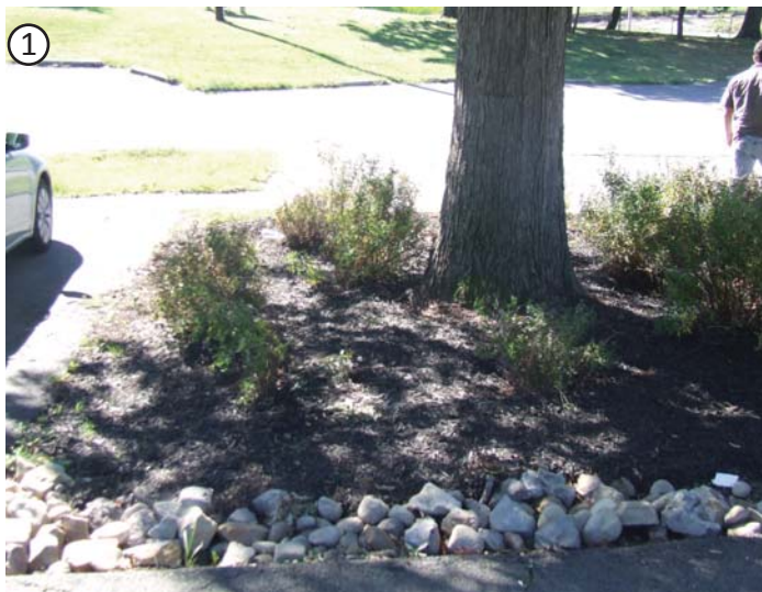
1 A small rain garden has been installed in an existing gap in the parking lot.
